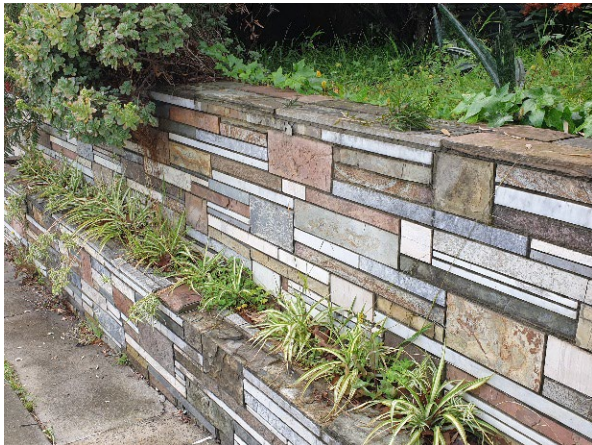
Figure 8 Section of fence/retaining wall with integrated planter on lower level. (Source: GML 2021)
