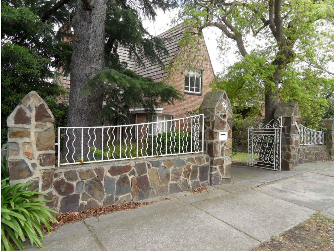
Figure 4. The early masonry front fence with mild-steel infill and gate. (Source: Context 2017)
